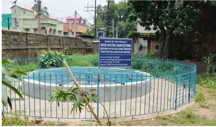
Rain water harvesting (ground water recharge circular shaped trough injection well)
